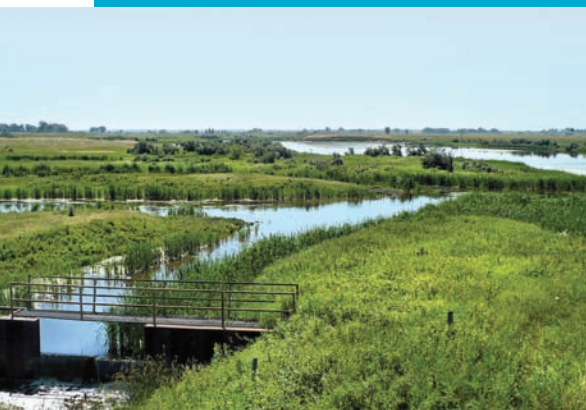
Landowner management agreements include the installation of water-control structures, like this one near Patricia, Alberta./©Ducks Unlimited Canada
