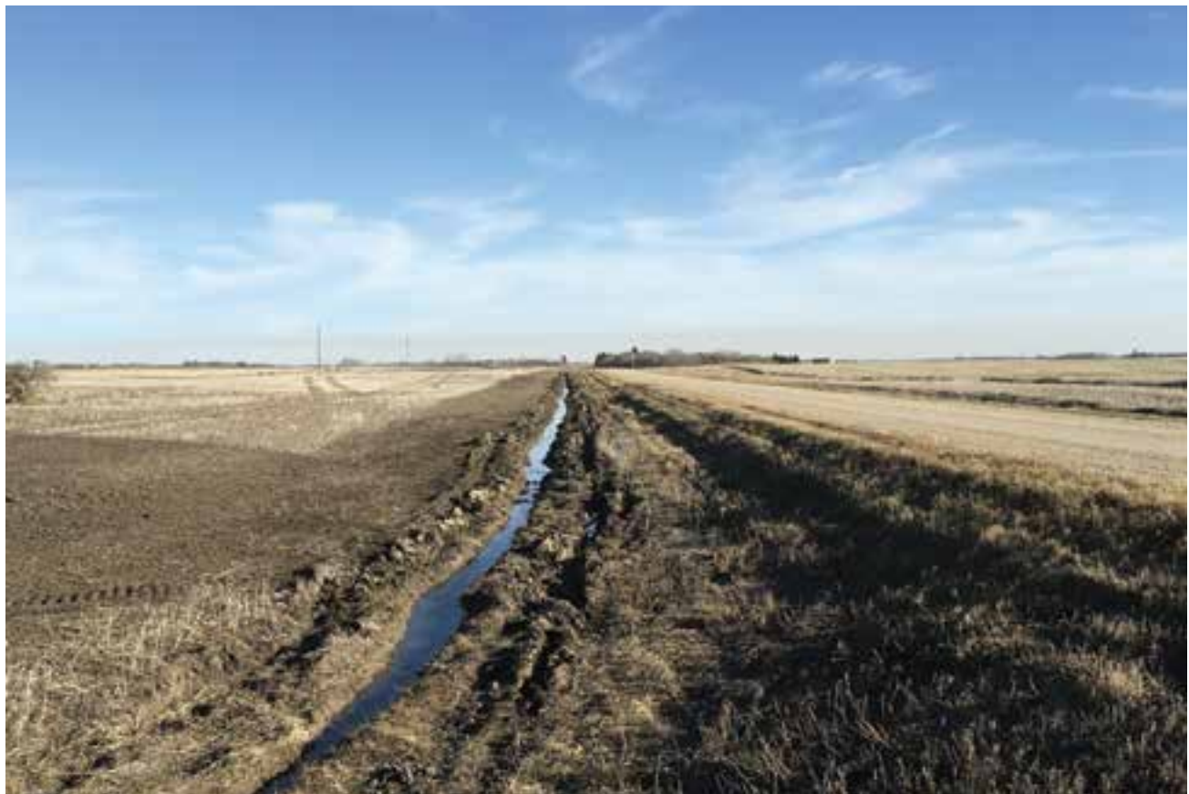
Figure 12. An example of a roadside ditch being utilized for consolidation and transport of drainage water.
