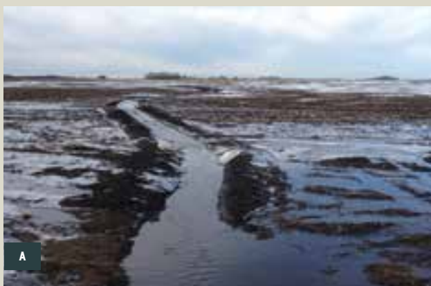
Figure 16A (left) & 16B (right). (A) Shows a fall constructed ditch targeting multiple wetland areas draining early spring melt water. (B) The same area as shown in image (A) later in the spring of the same area during seeding. Note how the ditch has been removed from the landscape and all the spring runoff has been drained from the field. This seasonal drainage technique can thus be very difficult to quantify and detect.
