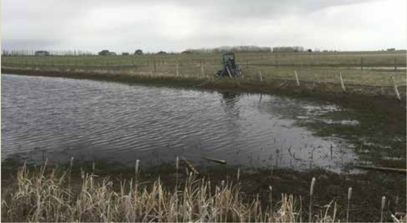
Figure 17. An example of a motorized pumping system being utilized to draw down a spring flooded emergent deep marsh habitat.
