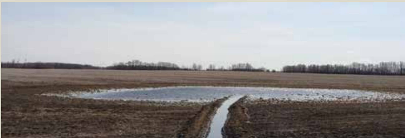
Figure 15. An example of a fall constructed ditch draining a seasonal type wetland and consolidating drained water in the roadside ditch.
